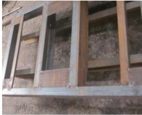
Figure 1: Steel Platform Structure
