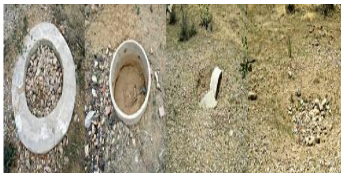
Figure 9: Rain Water Recharging Pits at Kaladera.
