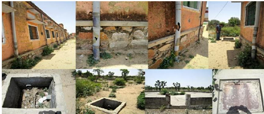
Figure 7: Rain Water Harvesting Plant at Government School at Kaladera.
