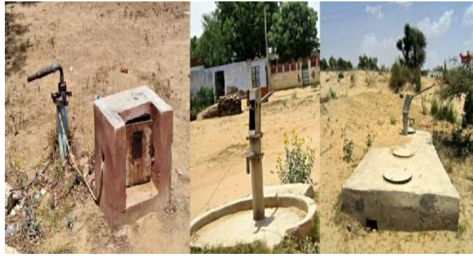
Figure 10: Bore Well and Hand Pumps at Kaladera.
