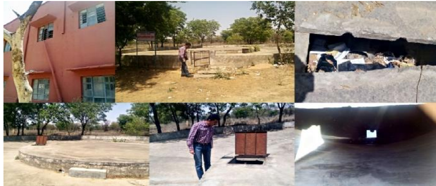
Figure 6: Rain Water Harvesting Plant at R.L Sahariya College at Kaladera.
